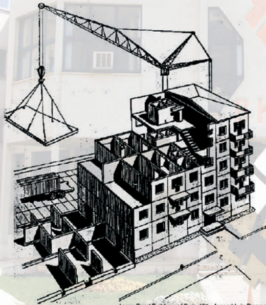
Largo Panel Buildings of Siria 135 - Assembly in Progress
